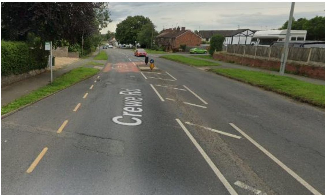
Pedestrian refuges at controlled crossings
