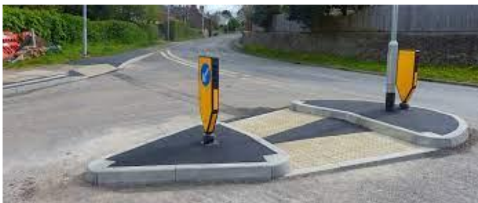
Figure 2 Example of a dropped kerb with a pedestrian refuge
