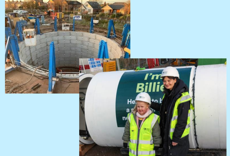
Delivering upgrades to the local sewer network in Cottam, Preston
